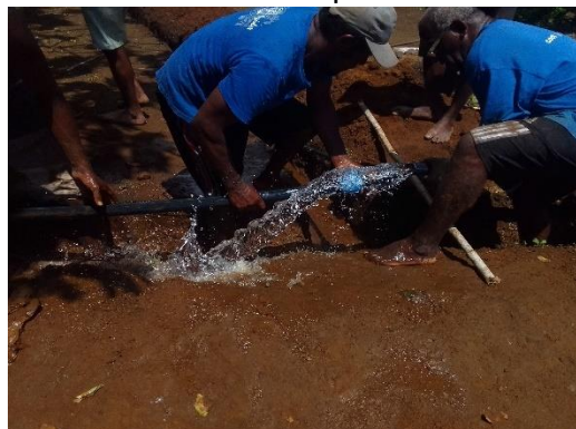
Figure 3: Distribution Pipe installation at Lalnetak village, Vanua Lava
