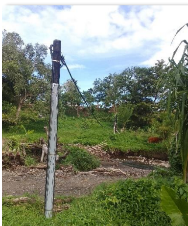
Figure 4: Support structure for creek crossing overhead line between Lorlow and Wintua village damaged by TC Kevin & Judy in March 2023
